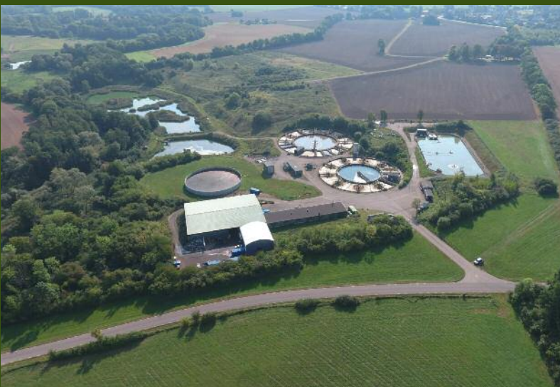
View of the industrial process treatment plant in Bjuv, Photo: Bengt Fellbe
